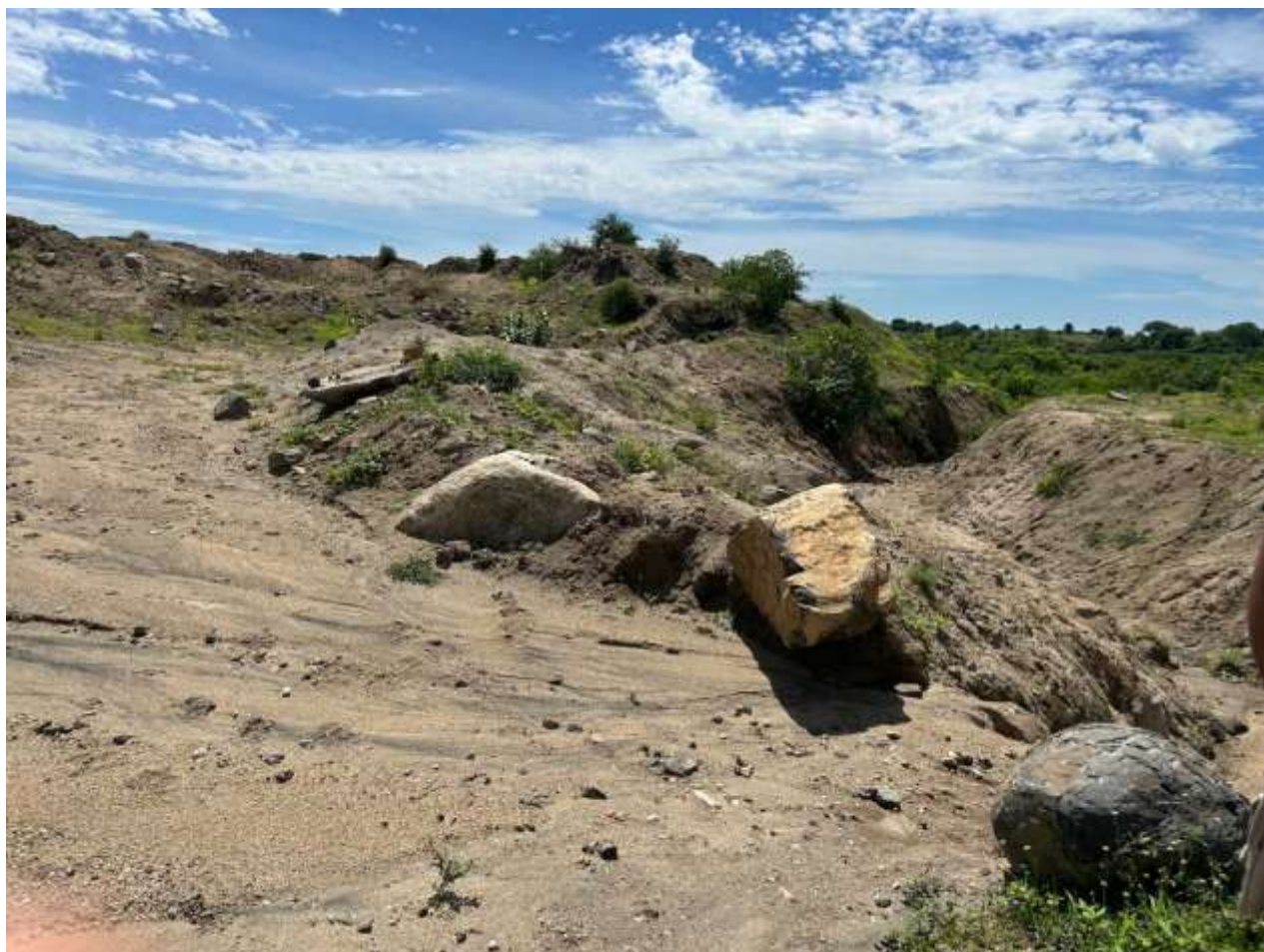
Natural channel at siphon 5
