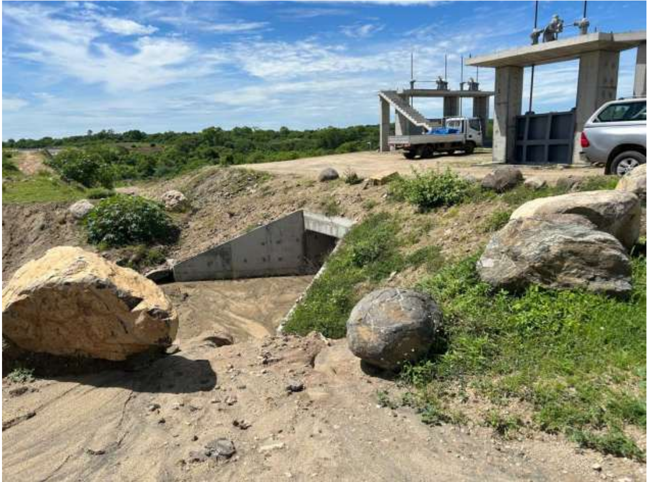
Proposed site at siphon 5
