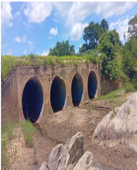
Siphon 3: Downstream Majete road (T416) culvert washing clothes
